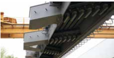
Craned MAURER Swivel Joist Modular Joint
