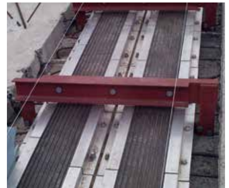
Installation of MAURER Double Mat Joints
