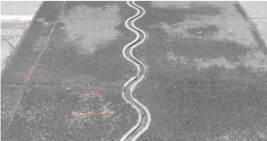
Donnersberger Bridge, Munich / Germany
