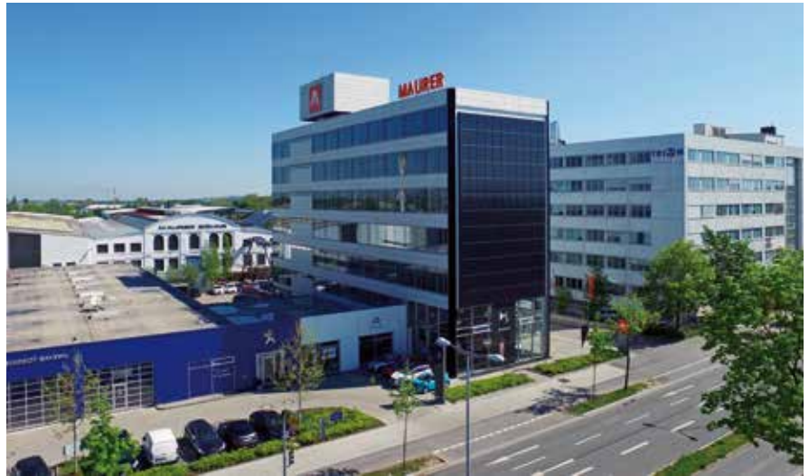
MAURER headquarters, Munich / Germany
