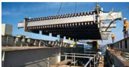
MAURER Swivel Joist Expansion Joints
