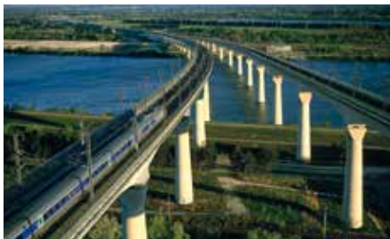
TGV railroad section near Avignon / France
